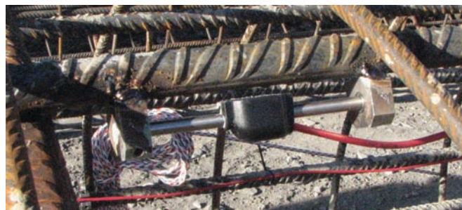
Figure 1b. Strain gage embedded in concrete.
